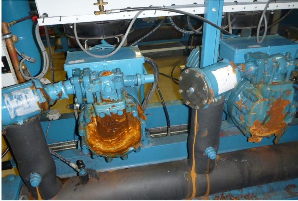
**FIGURE 18.** EXAMPLE OF A HIGHLY CORRODED COMPRESSOR FLANGE
