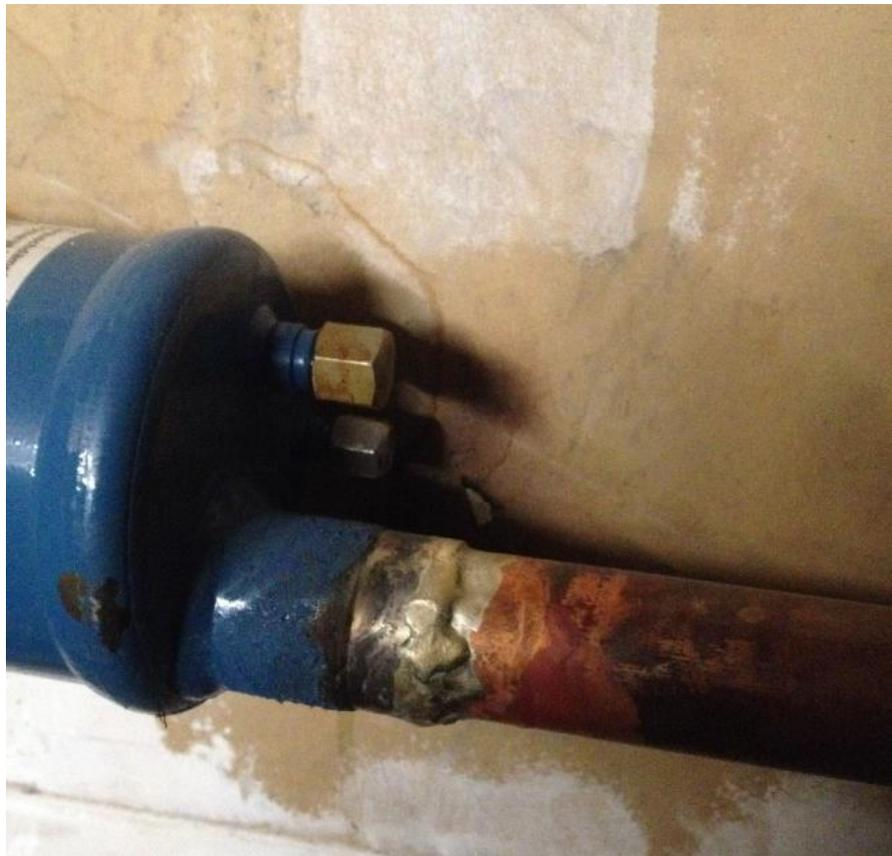
**FIGURE 21.** EXAMPLE OF A POORLY PERFORMED WELD
