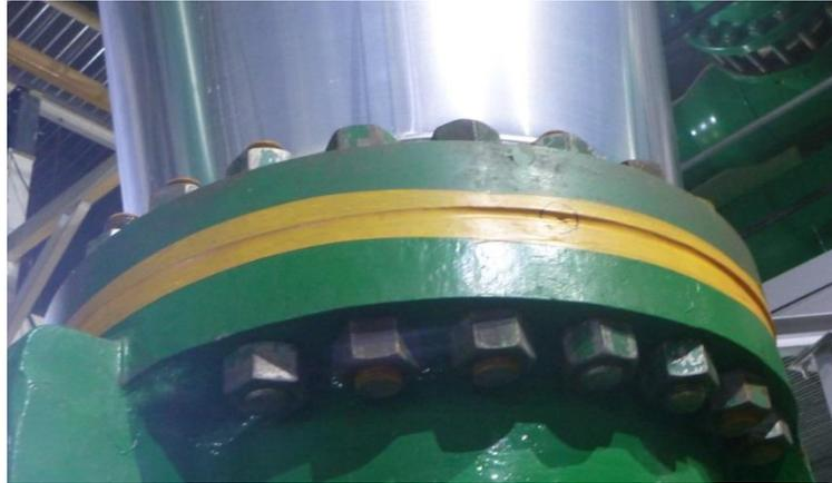
**FIGURE 24** EXAMPLE OF CAULKING A FLANGE FOR MORE EFFICIENT LEAK DETECTION
