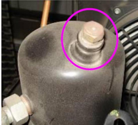
Fusible plugs: wide temperature and/or pressure variations weaken the bond between the core and the plug
