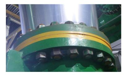
FIGURE 24 EXAMPLE OF CAULKING A FLANGE FOR MORE EFFICIENT LEAK DETECTION
