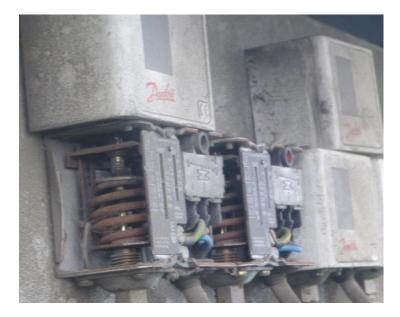
FIGURE 20. PRESSURE SWITCH WITH NO PROTECTIVE BOX, PRESSURE SWITCH BELLOWS IN BAD CONDITION
