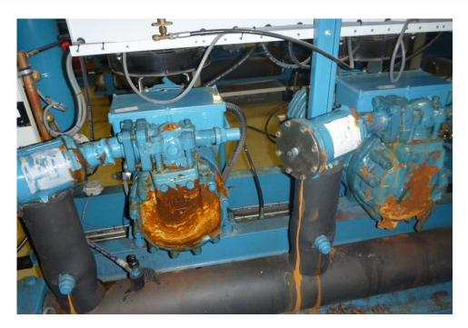
FIGURE 18. EXAMPLE OF A HIGHLY CORRODED COMPRESSOR FLANGE
